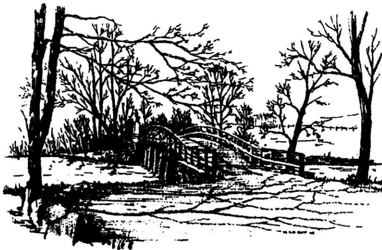
Old North Bridge, Concord, Massachussets
